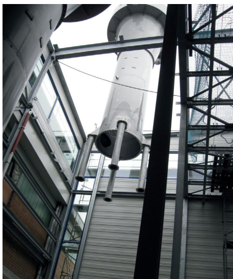
Installation of the softening reactor
