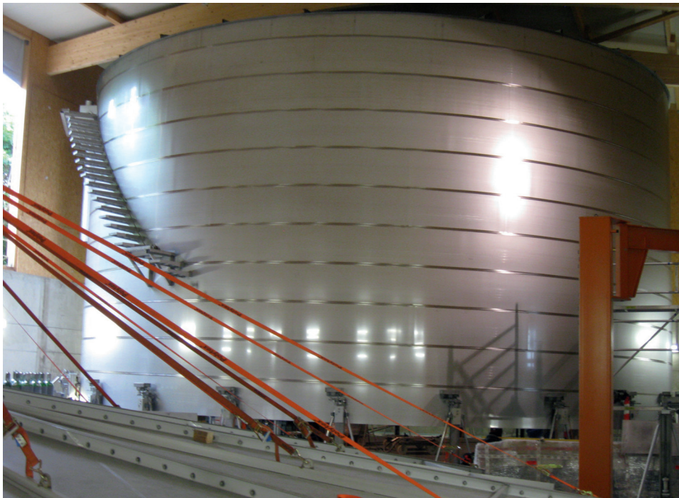
Manufacturing of the drinking water storage tank made of stainless steel 304 in Haar near Munich
