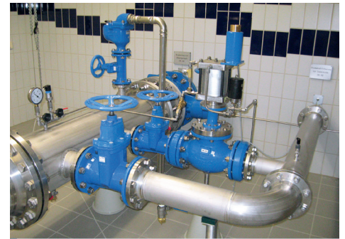
Overpressure protection with special valve
