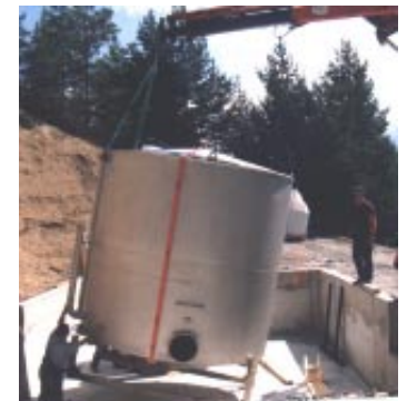
Fig. 3: Installation of the Hydro-Clear
