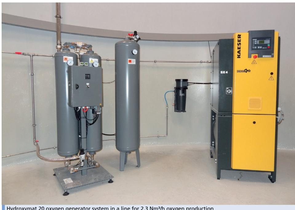
Hydroxymat 20 oxygen generator system in a line for 2.3 Nm<sup>3</sup>/h oxygen production
