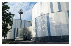
stainless steel tanks 15.75 metres in diameter and with a capacity of 1500 m<sup>3</sup> each were set up initially, before being integrated into the system both electrically and hydraulically. The tank system with its state-of-the-art air filtration technology was
