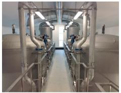
The system is constructed in two entirely separate lines and was designed for a treatment capacity of 80 m³/h. The process steps are CO2 enrichment - ozonisation – contact column (D = 1300, H = 6000 mm) - hardening via marble filter (D = 2500, H = 4000 mm) upstream - multilayer filtration (D = 3000, H = 4000 mm) for bio-filtration and particle separation downstream - UV radiation.
