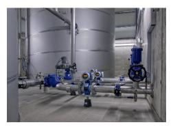
The complete stainless steel tank system (duplex steel) with the associated electrical and hydraulic V4A stainless steel installation and the conversi-
