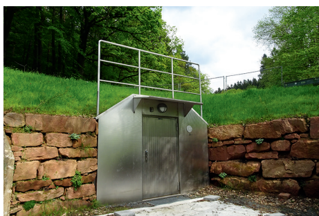
Access to the pumping station
