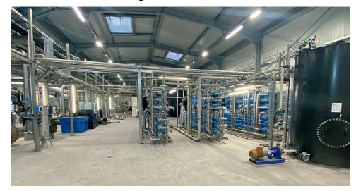
Teamwork within the HydroGroup® resulted in a condensate cleaning system (CCS) for treating the reflux condensate.
