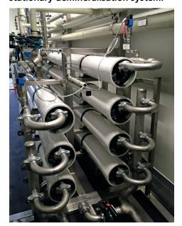
The ultra-pure water trailer reliably produces 20 m³/h of deionized water in VGB ultra-pure water quality. The rarely-required changing of the filter cartridges and a process chemicals refill interval of a few days mean that the customer's staffing costs are low. In addition, maintenance work by RWT for mixed-bed filter resin changes is very seldom required thanks to the oversized mixed-bed filters.
