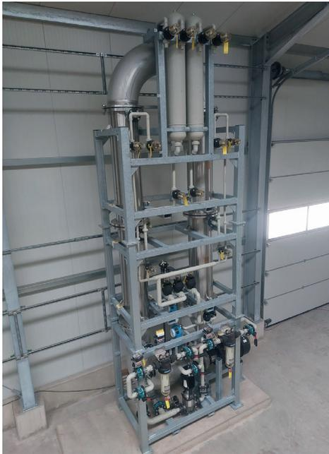
**Problem:** condensate cannot be discharged into the wastewater sewer without prior treatment due to high concentrations of dust (particle load), ammonia or ammonium, and dissolved organic substances with a high vapour pressure. This is why RWT GmbH was commissioned to plan and construct an exhaust vapour condensate treatment system.
