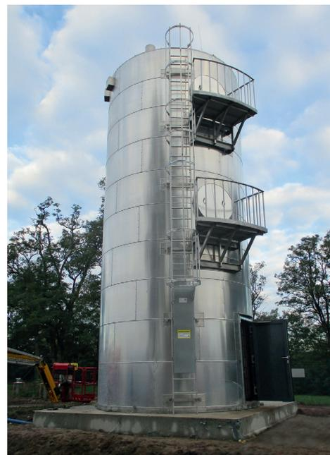
One HydroSystemTower® with a volume of 2 x 30 m<sup>3</sup>, an integrated pressure booster system, extensive installation and a control system was manufactured, moved to its installation site and commissioned to supply water to a military training area in eastern Germany.
