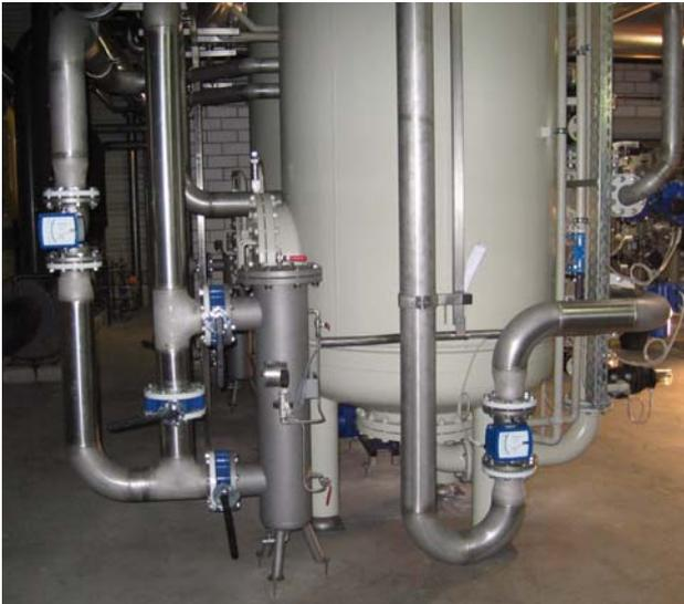
Condensate polishing line with resin trap
