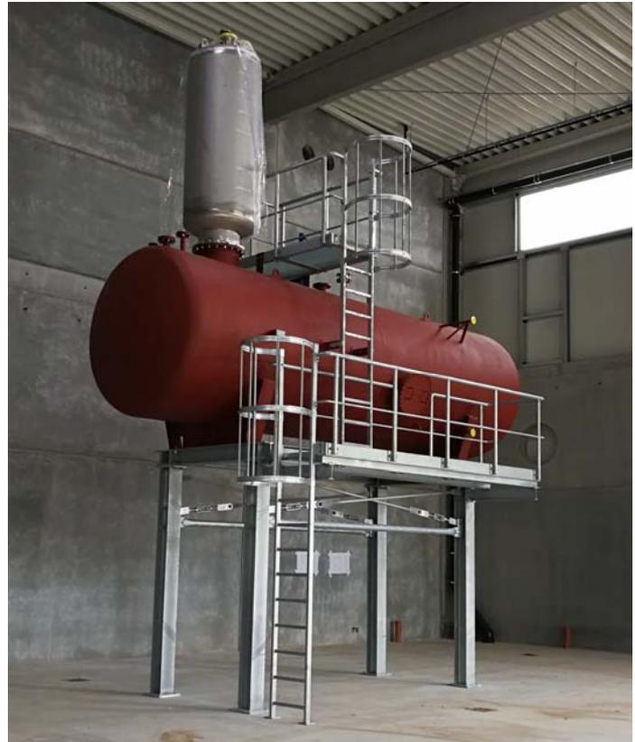
Degasification after erection
