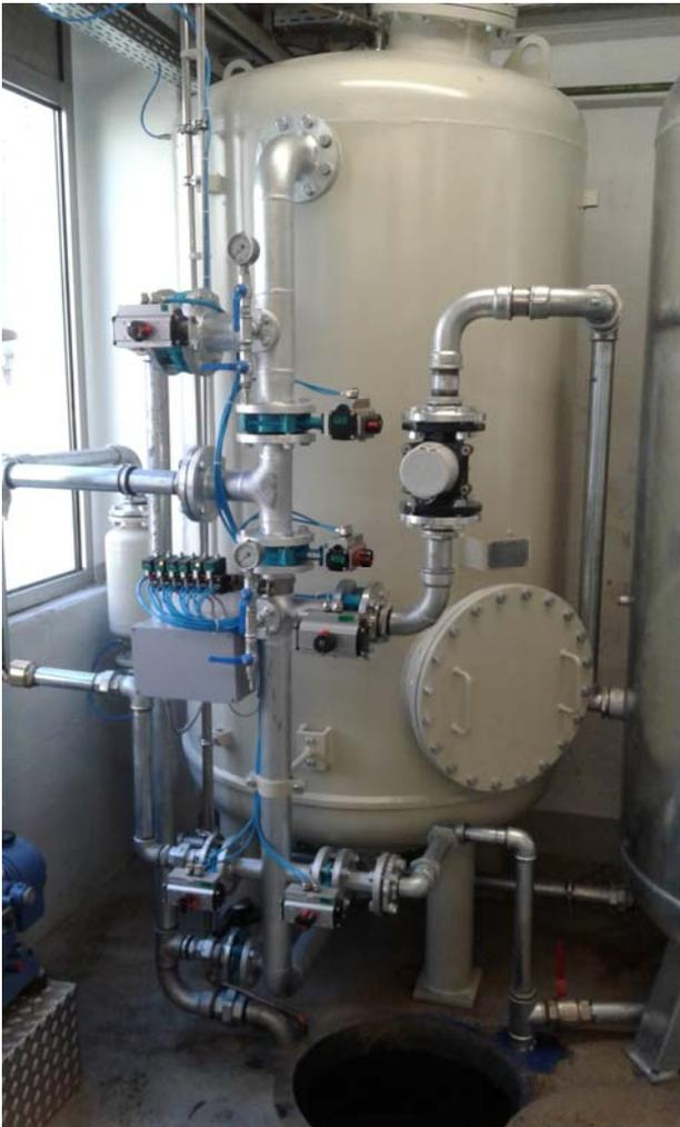
Filter vessel with automatic front piping
