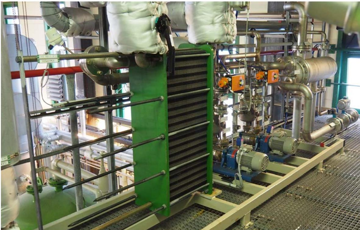
Rack with vapour condenser, vacuum pumps and additional preheater for feed water (from right to left)
