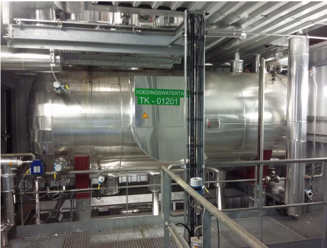
Degasification plant after installation and insulation by customer
